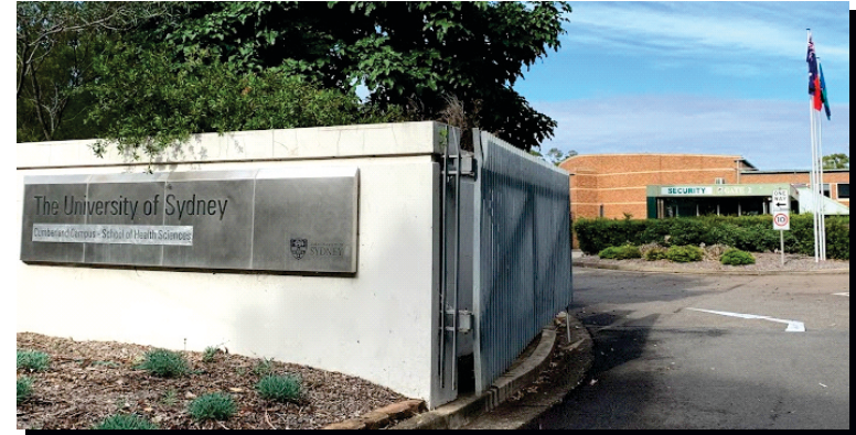
Photo of the abandoned University campus on East St, a good site for the new Lidcombe High School/ Public School and Early Education Centre of Excellence.
